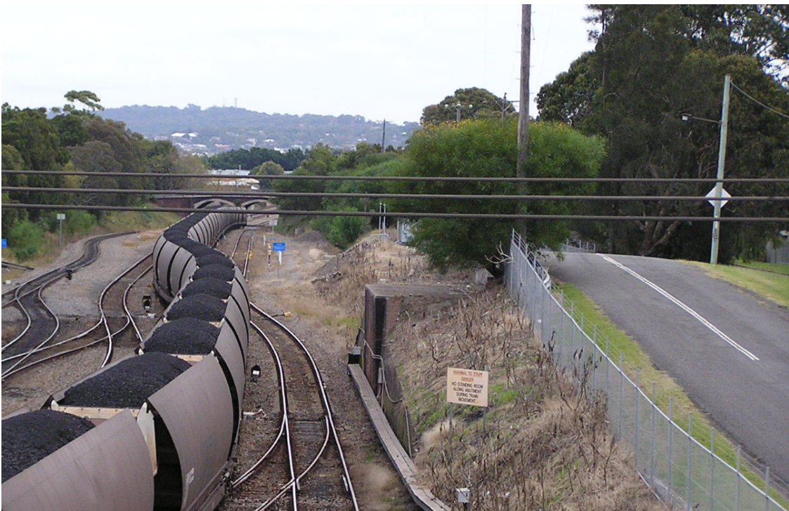
Figure 8 - May 2008 photograph showing the remaining western approach embankment and abutment of the former Rose Street overbridge. Source: Sam Laybutt.
