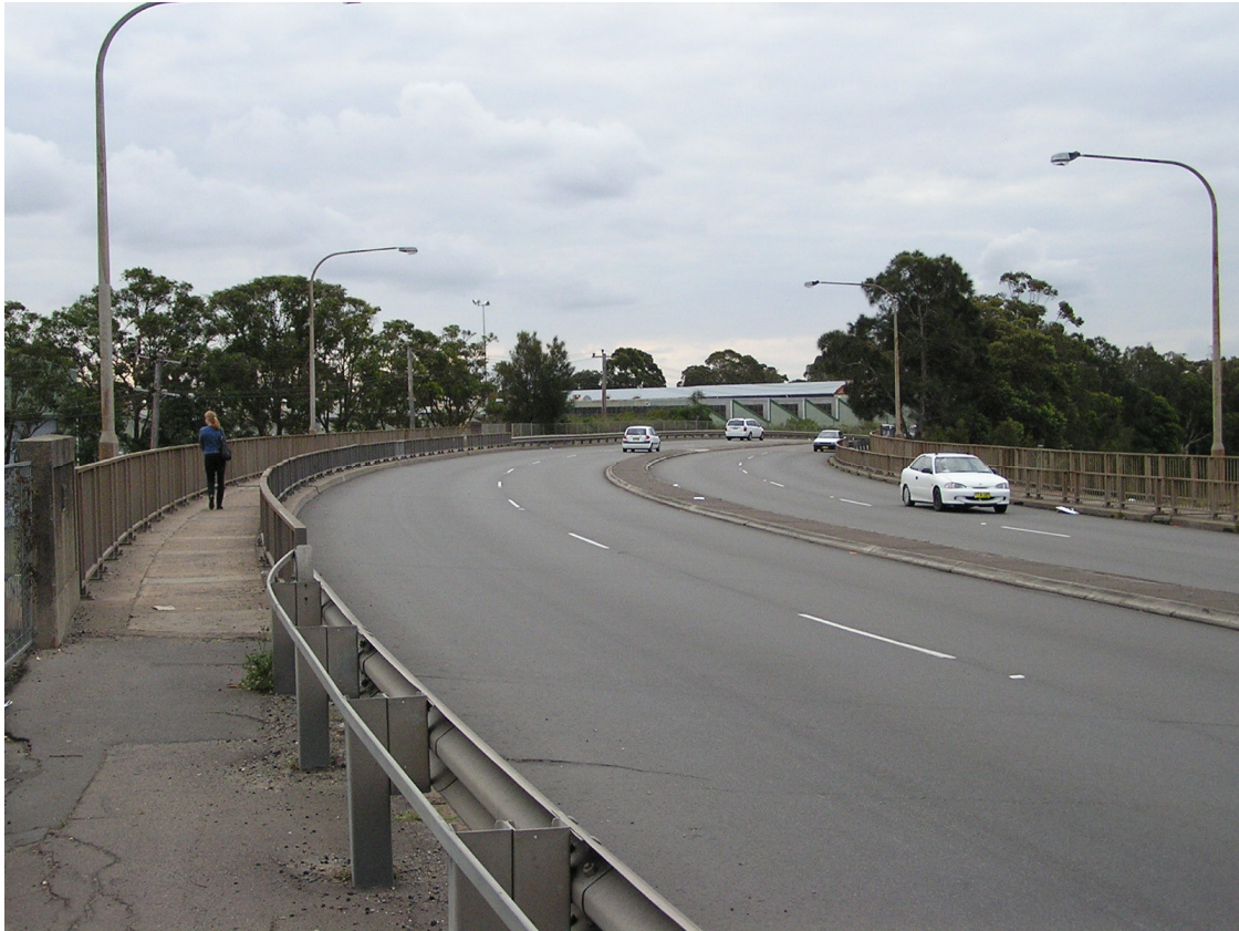
Figure 6 - May 2008 photograph showing the bridge carrying Industrial Drive over the Port Waratah railway line. Source: Sam Laybutt.
