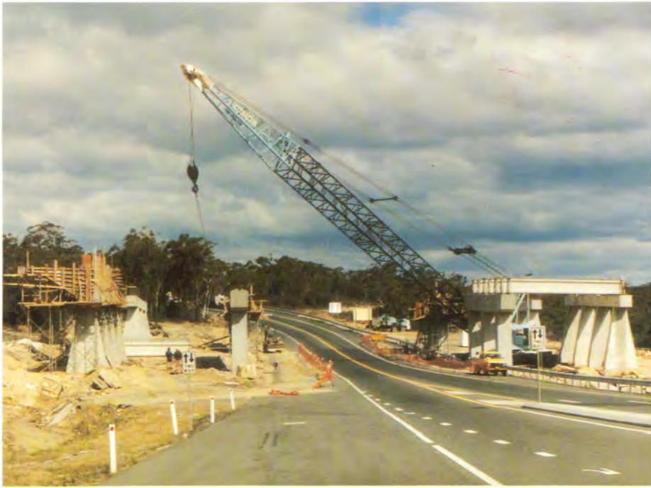
Pacific Highway access was maintained during the building of these bridges at Kariang Interchange.
