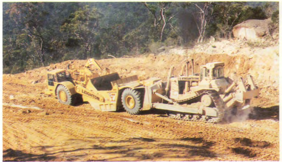
Construction contractors used some of the largest earthmoving equipment available in Australia.
