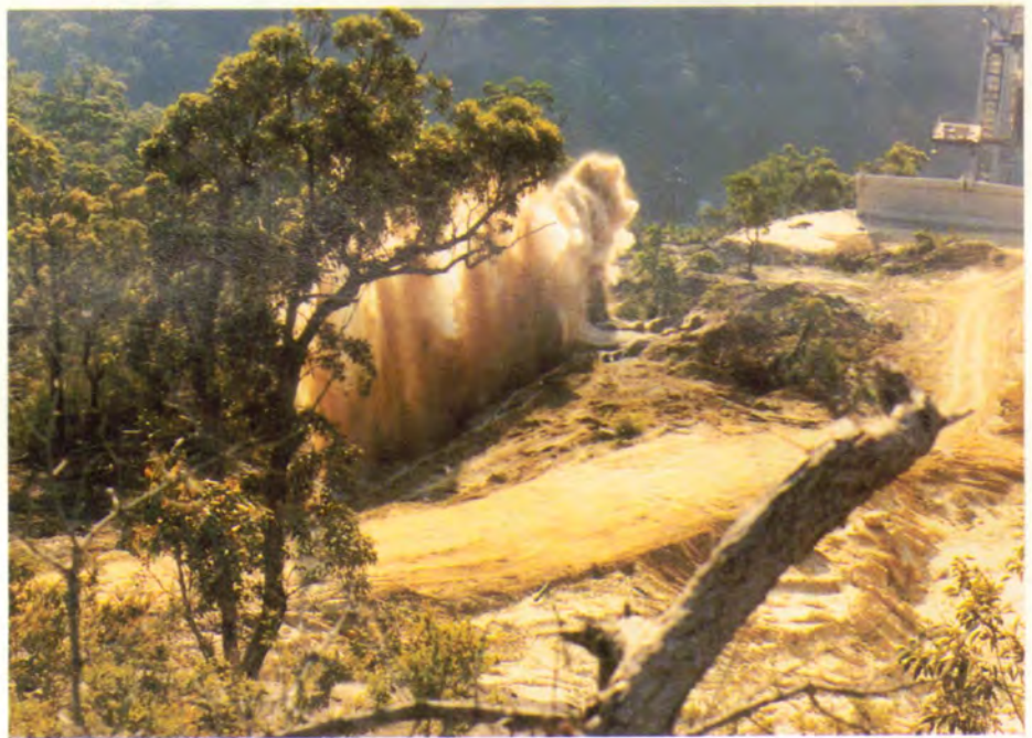
Careful blasting and earthworks operations ensured minimum effect on the natural environment.
