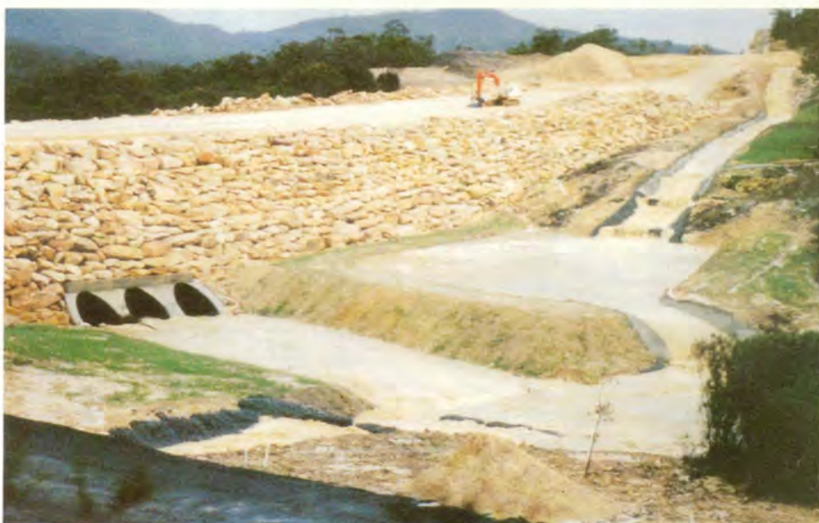
Above: Heavy rains during the construction period tested these erosion and sediment control works adjacent to Leask Creek.
