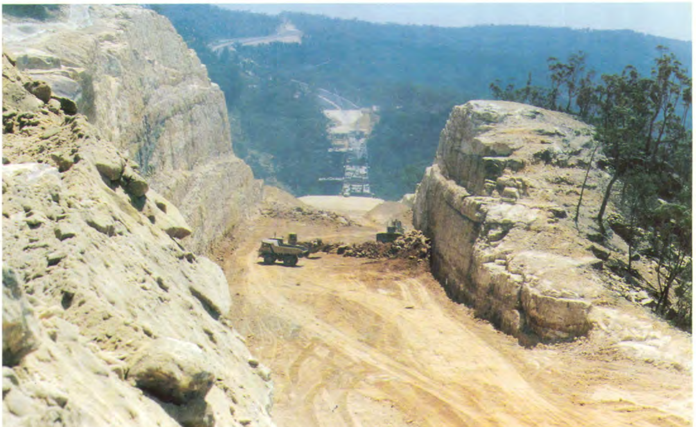
The deepest cutting (40 m) on the project is just east of Mooney Mooney Creek.
