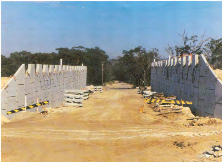
Reinforced Earth walls form the abutments of the twin freeway bridges over Gindurra Road.
